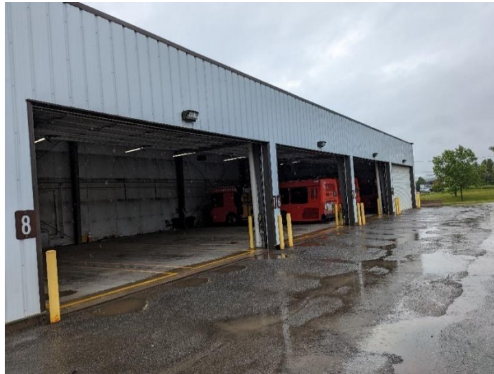
Figure 6 Bus Bay "Warm Storage" Area
