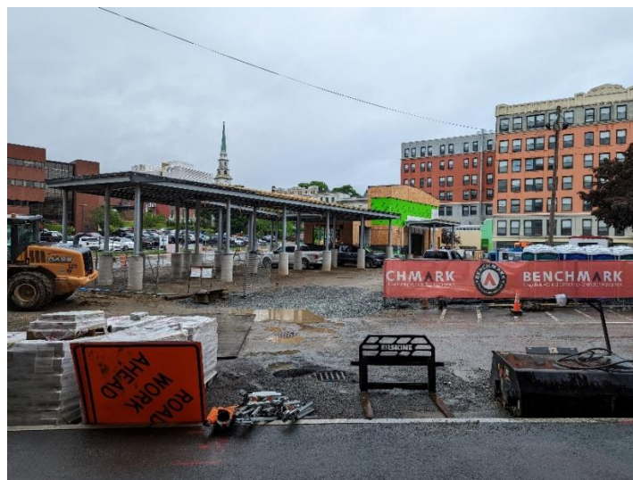
Figure 9 Pickering Square Transit Center Under Construction (June 2022)
